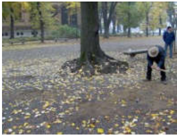
1a) Excavation around healthy trees in a selected environment
