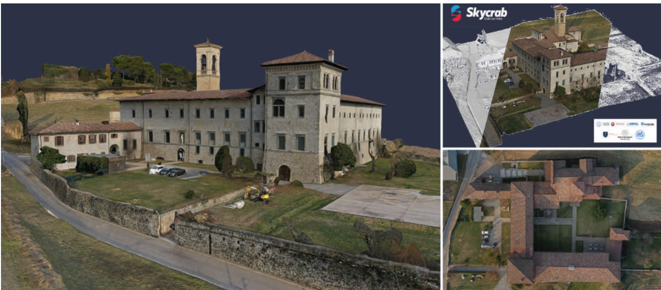
Figure 8. The as-built survey of the convent undertaken in 2019: DJI® Mavic-2 PRO drone, processing with CapturingReality® Reality Capture. (with @Skycrab Academy)
