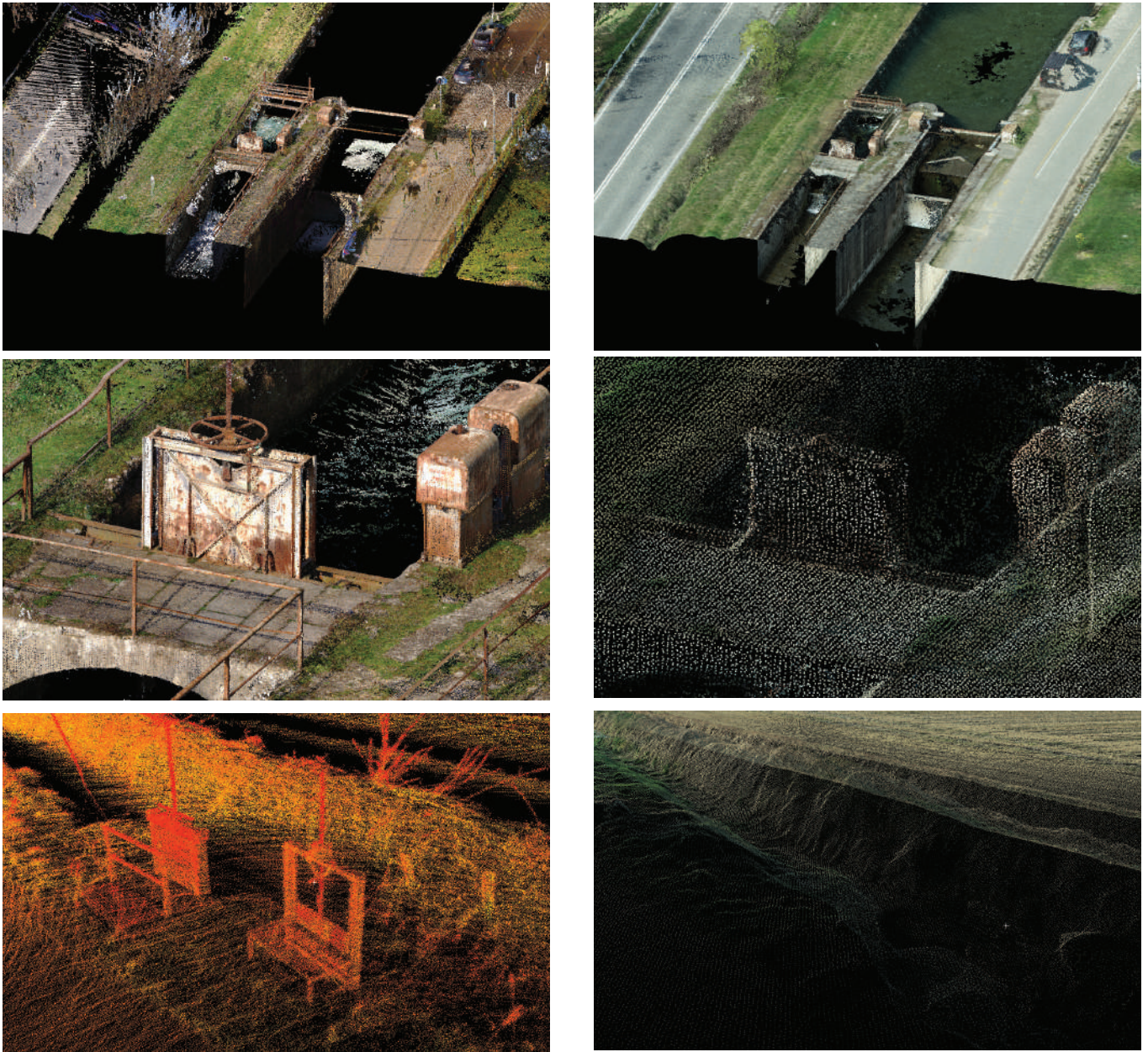
Figure 10. On the left: Terrestrial and Mobile laser scanner for the definition of territorial, architectural and detailed elements of the Naviglio Pavese. On the right: UAV's point clouds, with different levels of detail from territorial to architectural elements.
