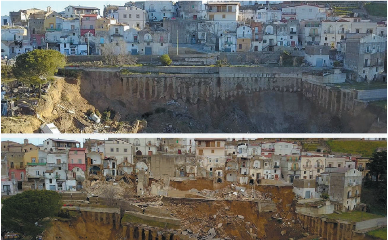
Figure 6. Pomarico: drone photos before and after the landslide.
