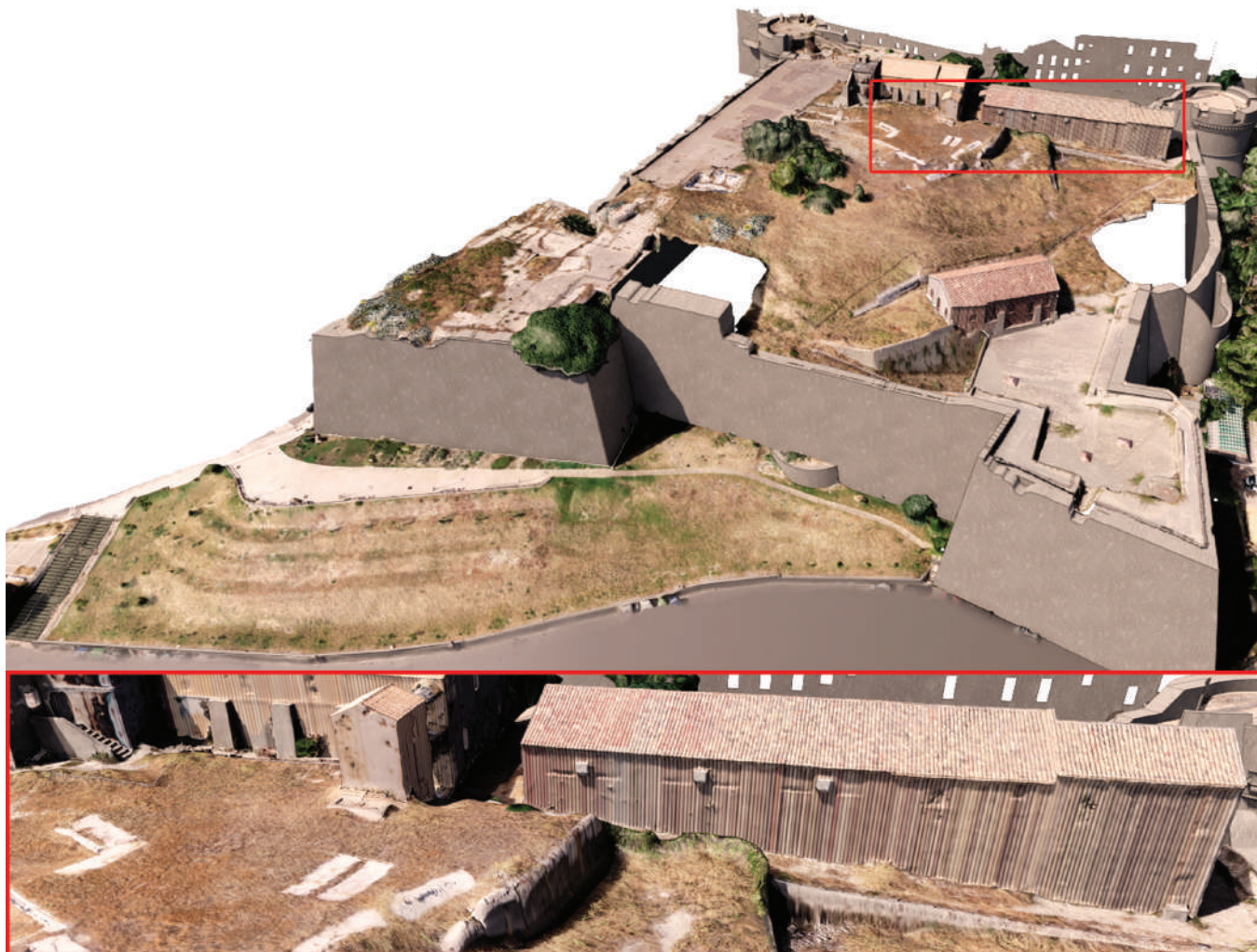
Figure 7. Results of the workflow A with evidence of texturing defects in vertical elements.
