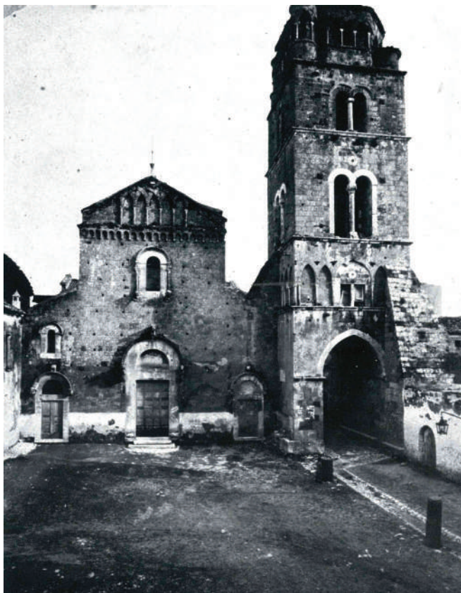
Figure 2. Historical photograph of the bell tower before the restoration of 1960-1963. Source: M. D'Onofrio, The cathedral of Caserta Vecchia.
