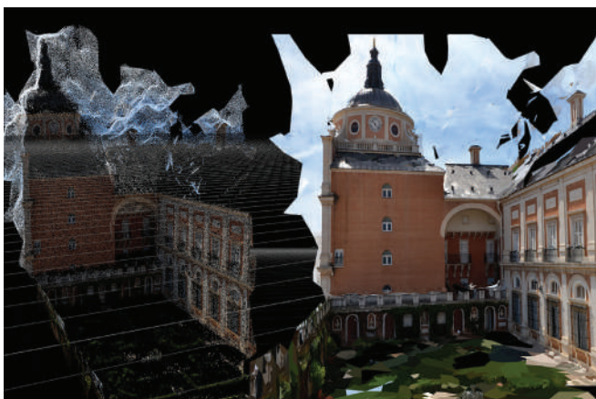
Figure 9. Royal Palace of Aranjuez, Eastward view of the courtyard of the King's private garden, from the dense point cloud to the processing of the precision orthophoto from textured mesh. (Gennaro Pio Lento, 2022)
