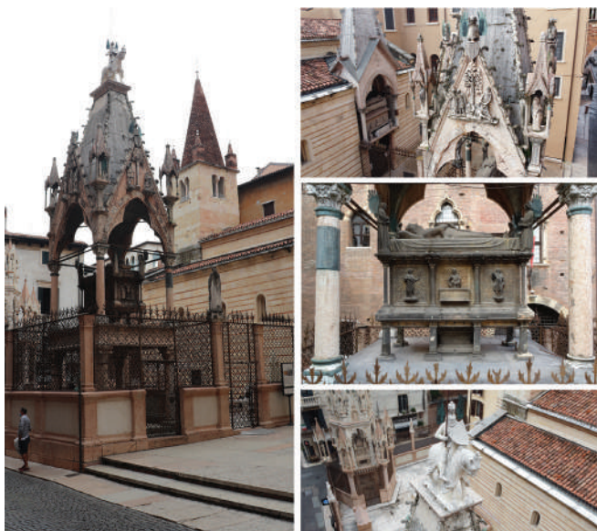
Figure 1. The Ark of Mastino II is made of marble and consists of two levels with a rectangular plan (approximately 3.10x3.50m) surrounded by marble columns, with a truncated pyramid roof. On the first floor is the sarcophagus, a remarkable sculptural work (1.25x2.45m) supported by a central pedestal and 8 small pillars at the sides. At the top of the monument is the statue of the deceased in civilian clothes, protected by four saints who are located inside the aediculae at the corners of the monument.
