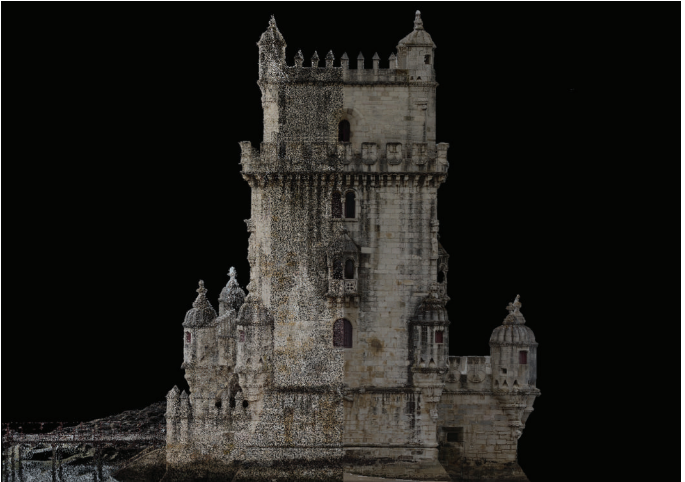
Figure 5. The Belem Tower in Lisbon. View of the main elevation of the dense point cloud and tex-tured mesh obtained through the photogrammetry process. (Guerriero Fabiana, 2021)
