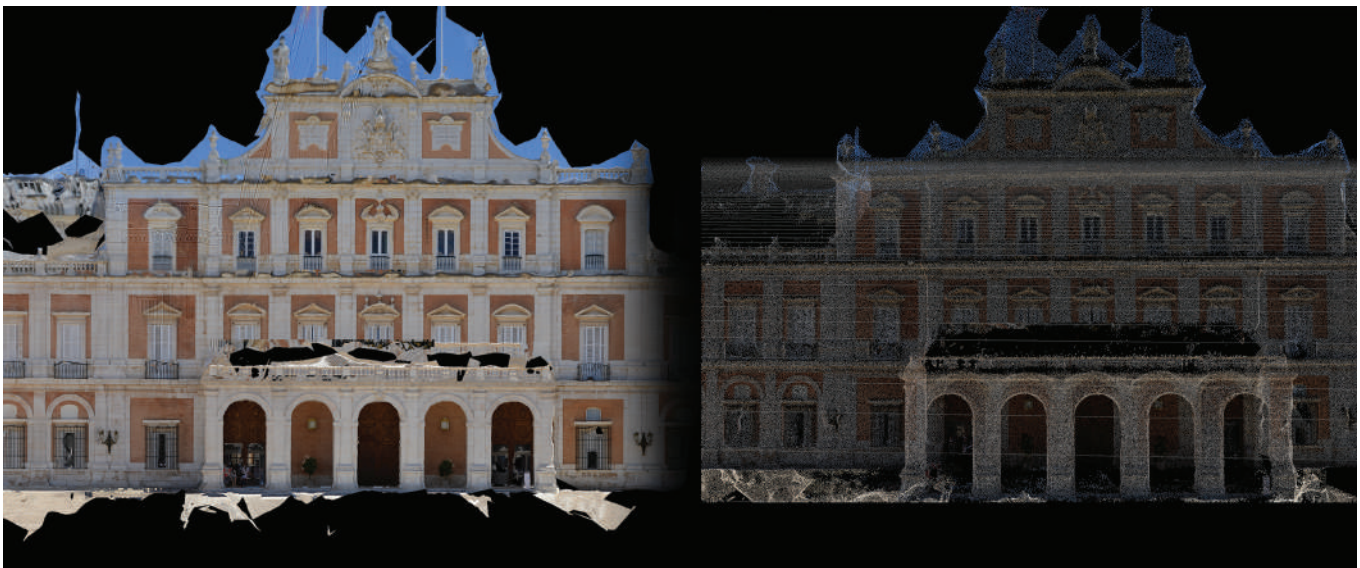
Figure 7. Royal Palace of Aranjuez, View of the main elevation, from the dense point cloud to the processing of the precision orthophoto from textured mesh. (Gennaro Pio Lento, 2022)
