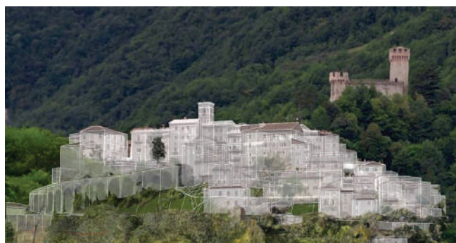
Figure 8. Arquata del Tronto: photo insertion of pre-seismic model (August 2016). (by M. D'Angelico)
