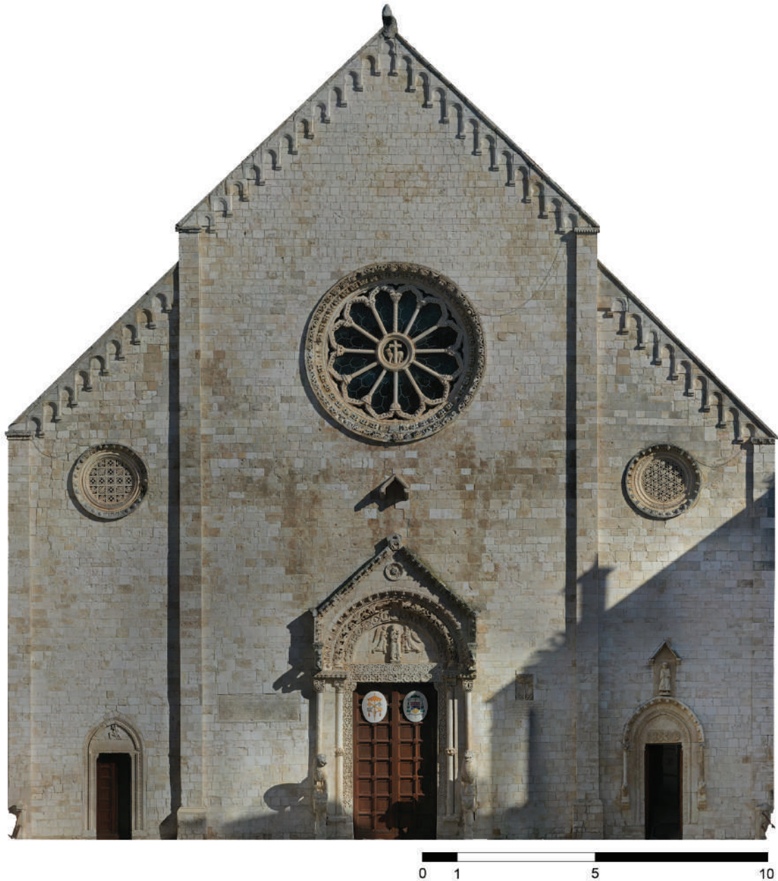
Figure 7. Photogrammetry of the main front Ovest.
