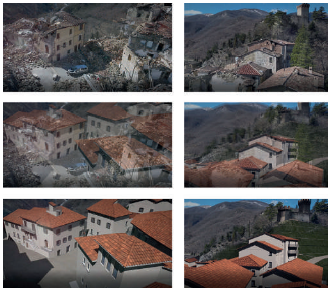
Figure 11. Arquata del Tronto: camera matching techniques for the reconstruction of buildings. (by M. D'Angelico)
