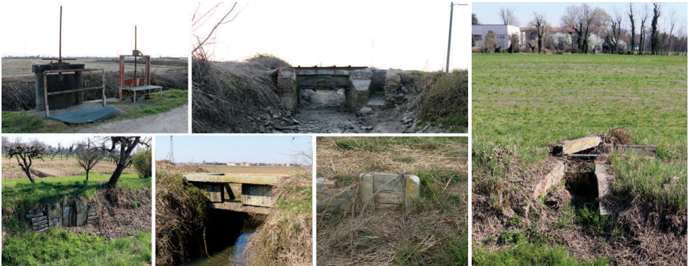
Figure 4. Elements of the irrigation systems.
