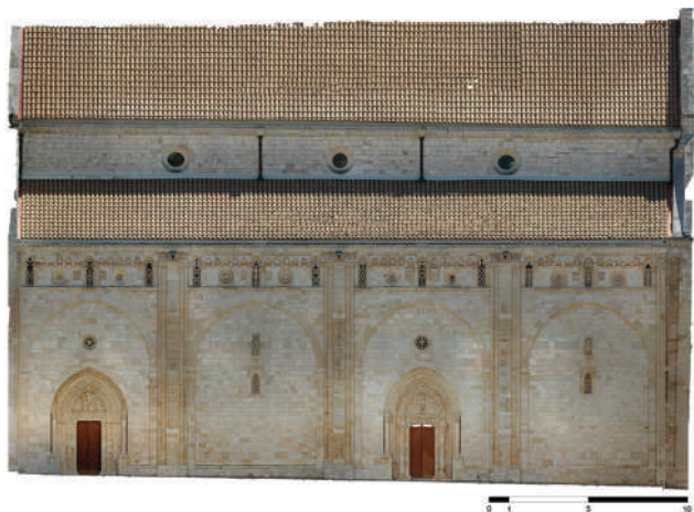
Figure 8. North elevation photogrammetry.
