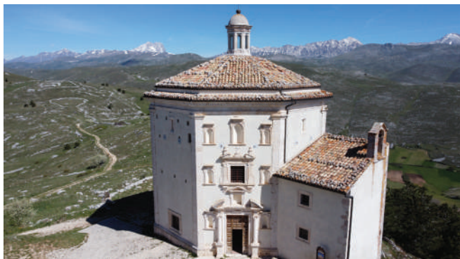
Figure 1. The main facade of the octagonal church of Madonna della Pietà; on the right the volume of the sacristy, in the background the Gran Sasso massif, with its highest peak, the Corno Grande, 2912 m asl.
