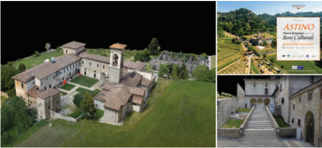
Figure 7. The as-built survey of the convent carried out in 2015: Dronica® MAP-1 quadrotor drone with Canon Eos M03 and 24 mm/1.4, processing with Pix4D® Mapper with @Dronica srl.
