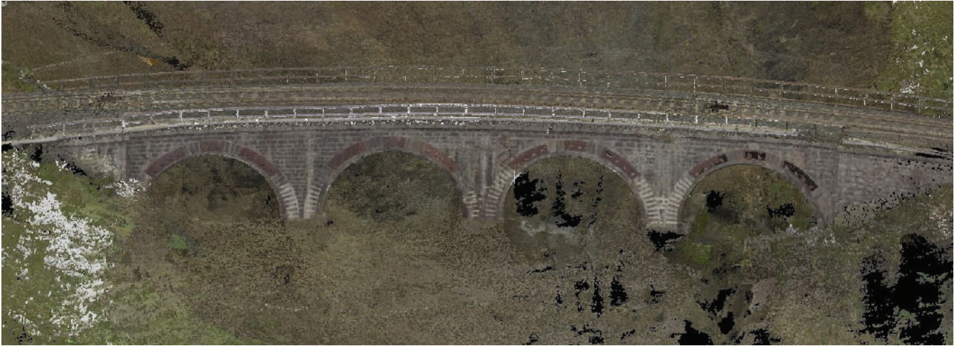
Figure 5. Point cloud obtained through TLS survey.
