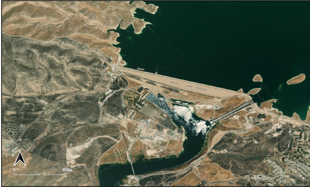
FIGURE 4 Bing Virtual Earth imagery of Mosul Dam site; notice the dam operation and the huge anthropogenic impact on the surrounding landscape
