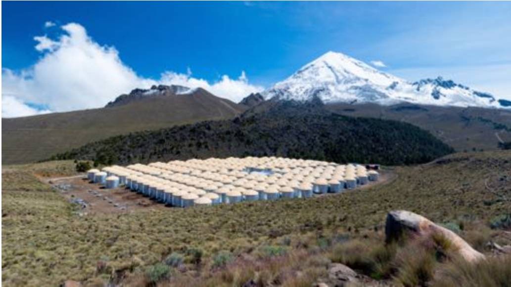
Fig. 1.10: Bird view of the High Altitude Water Cherenkov Experiment (HAWC), in 2014, Mexico. The full extension of 300 water tanks was completed in spring of 2015.
