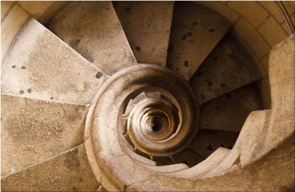
Spiral staircase inside one of the towers (A. Gaudí, 1925-1978, Sagrada Familia, Barcelona)
