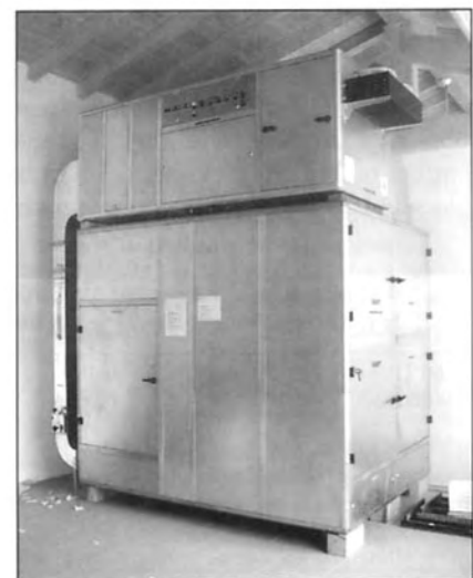
Fig. 1: Closed-circuit heat pump dryer (Valle Camonica, Italy) Abb. 1: Umluft-Kondensationstrockner (Lombardei)
