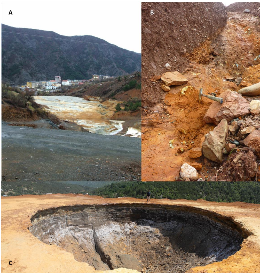
FIGURE 6: A - TAILING DUMP SHOWING MASSIVE SECONDARY PRECIPITATION AT FUSHE ARREZ (APR. 2015); B – WASHOUT IN R2 TAILING DUMP, REPS (NOV. 203); C –SINKHOLE IN THE ROOFTOP OF A TAILING DUMP AT KURBNESH (AUG. 2012)
