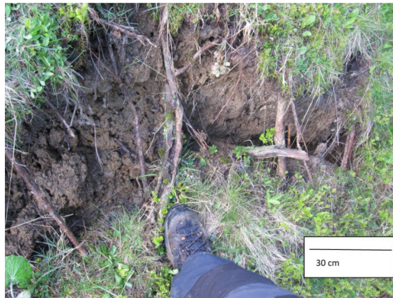
Fig. 3.2.3 Tension cracks in the 5 years old cutting area.
