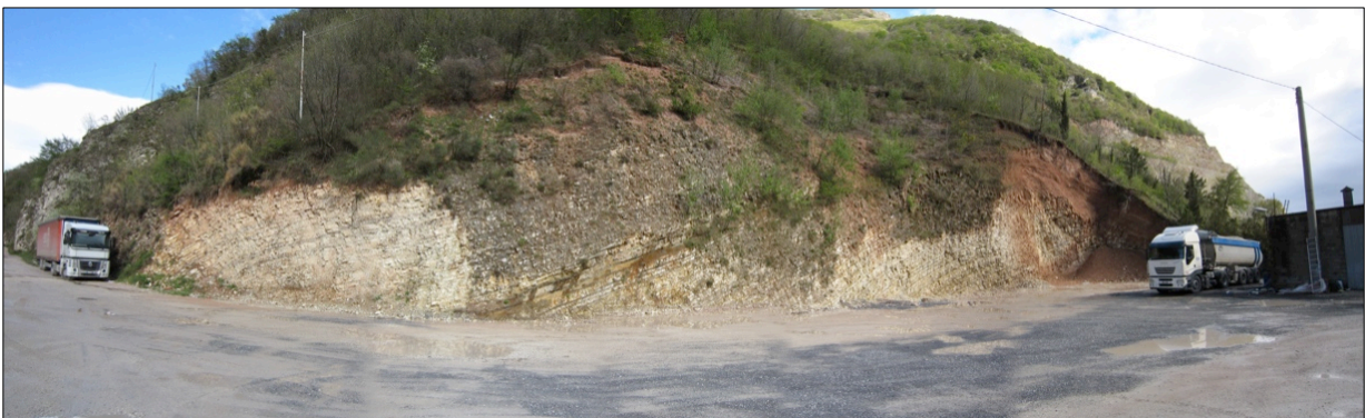
Figure 2.3a: Contessa section. The Gubbio2 core was drilled approximately where the truck on the left is located.
