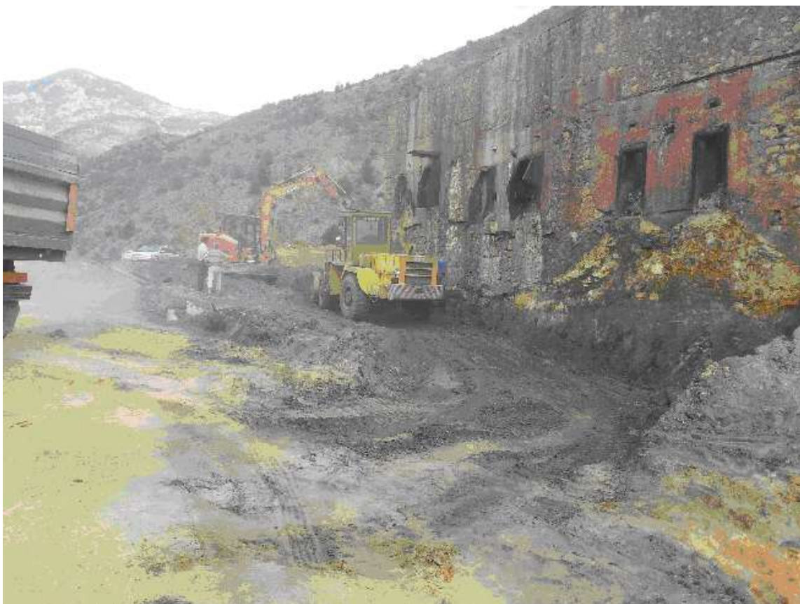
Fig. 61 Works after having loaded about half of the material.
