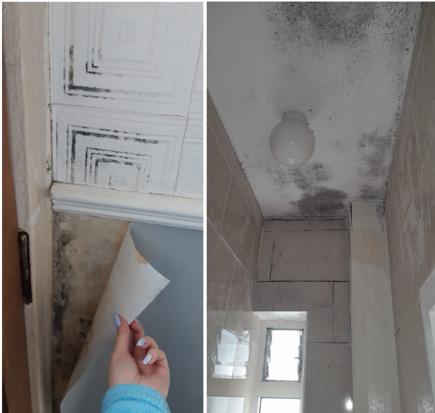
Figures 6 and 7. Mould in Oliver Bond House flats in the summer of 2022. Source: Photographs provided by residents.
