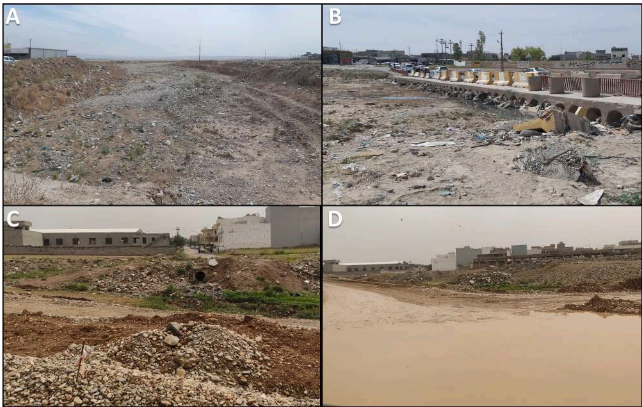
Fig. 9. A) A large valley crosses SE part of Erbil reworked by bulldozing. B) A blocked culvert, which led to overflowing of the valley during a heavy precipitation. C) A dumped valley in the eastern sector of Erbil city. Note the valley floor was transformed in paved road. D) A portion of the new ring road (R.R. 150) flooded during the 2021 event.
