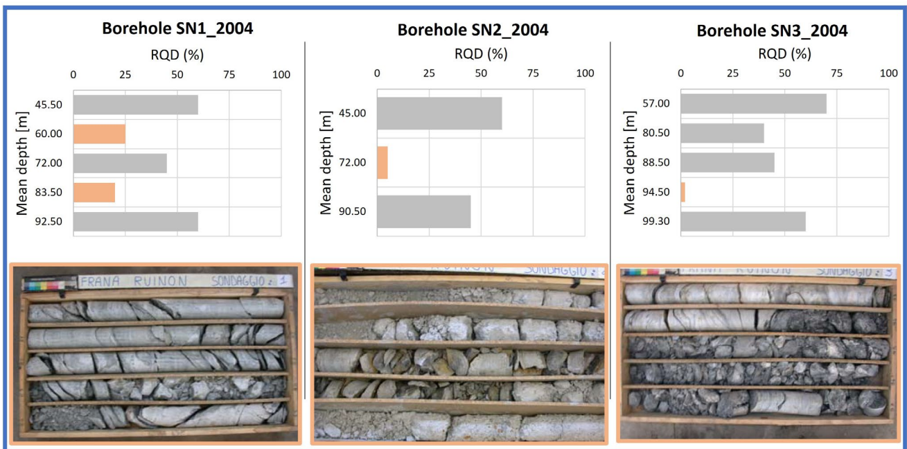
Figure 5.5 - RQD values measured at different depths in the boreholes SN1, SN2, SN3. The presence of heavily fractured layers is evident.
