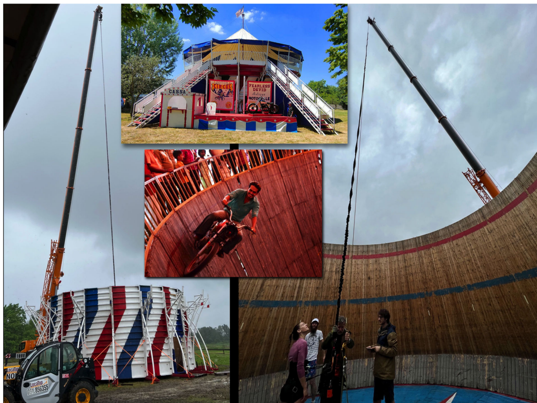
Figure 1. Top inset shows the WoD used in this investigation; left picture represents its ‘naked’ version, with the cap removed as to allow the telescopic crane to hang the body weight unloading bungee cords from a height of 36 m; right picture shows the vertical wall inside the WoD where horizontal running experiments took place at emulated (vertical) lunar gravity; middle inset displays a rider driving fast, with the peculiar upward leaning posture (see S2.5), during a WoD show.
