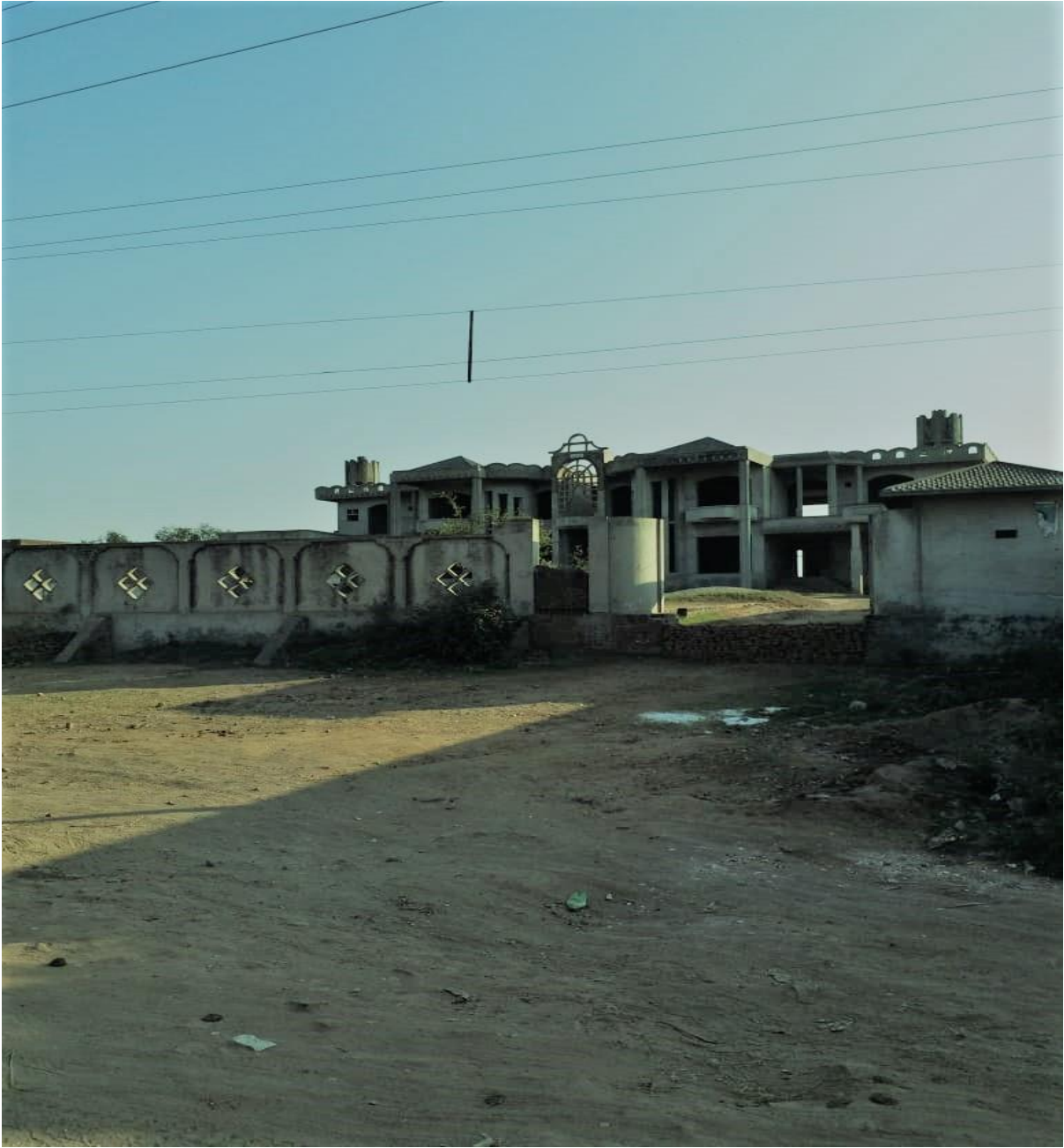
Photo sixteen: Under construction Kothi in the village
