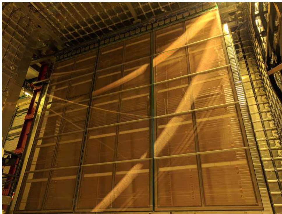
Figure 75: Three APAs installed and mechanically connected inside the cryostat.
