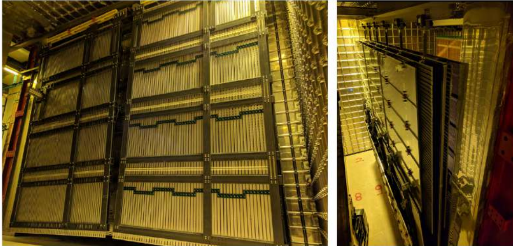
Figure 76: . Left: Salève-side drift FC end-walls are ready to be deployed inside the cryostat. Right: CPA and FC assemblies inside the cryostat ready to be pushed to their final position.
