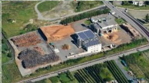
ORC unit of a Local district heating plant
