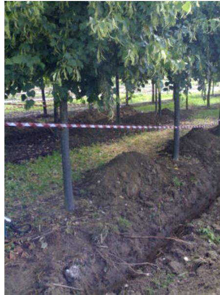
Trenching on 1 side of the tree - MD
