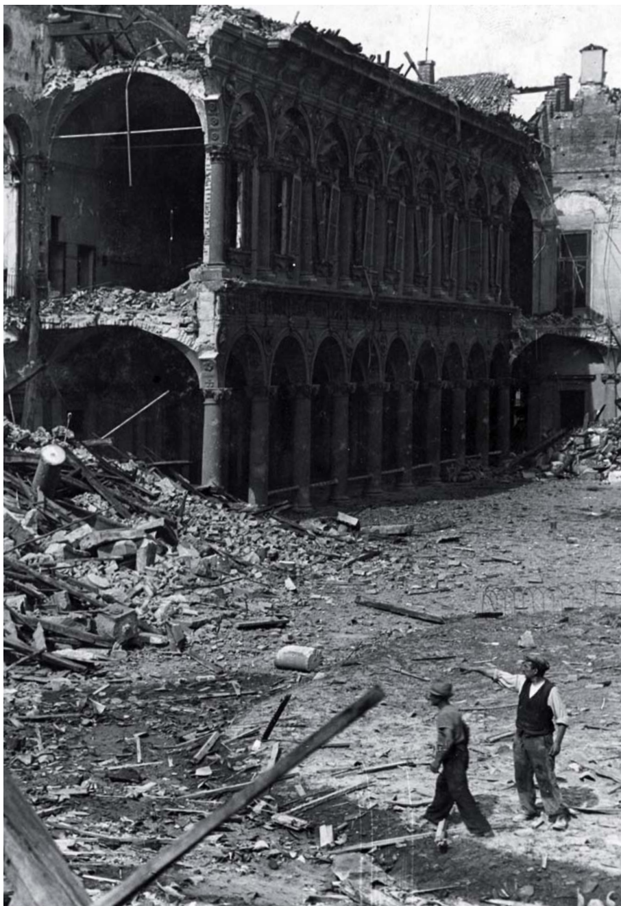
The serious damage caused by air raids in the Second World War, 1943. Milan, Archivio Ospedale Maggiore
