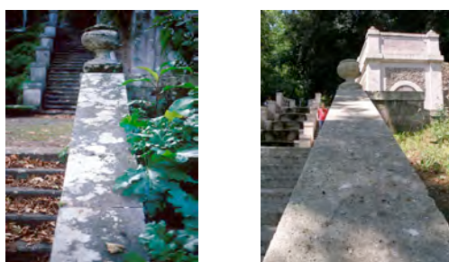
Fig. 1a-1b. Before and after restoration
