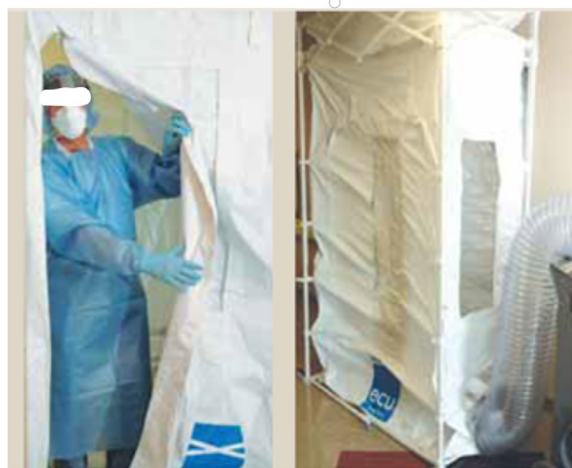
Figure 5. Temporary negative pressure isolation: although not as suitable as permanent ventilation solutions, a portable anteroom may be installed and connected to portable air ducts. Reproduced from public reference (7).
