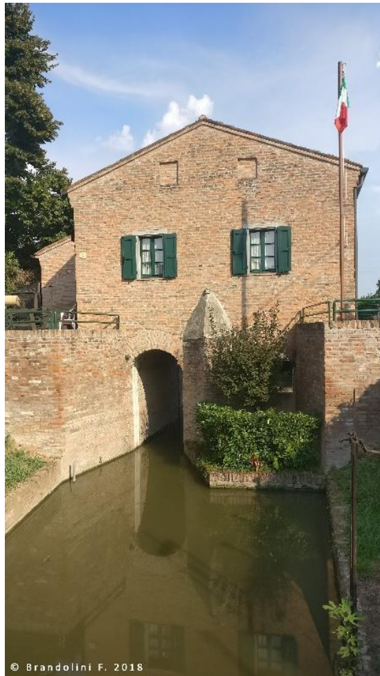
Figure 14. Medieval Hydraulic device on the Tagliata Canal. Point of interest n.3 along the Medieval geo-educational itinerary proposed.
