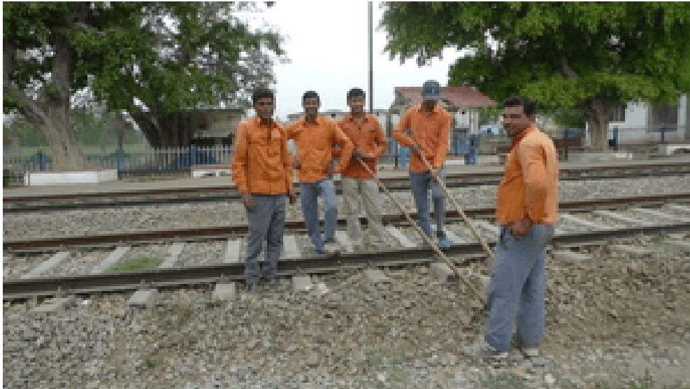
Figure A.21: Railway's workers in Palanpur
