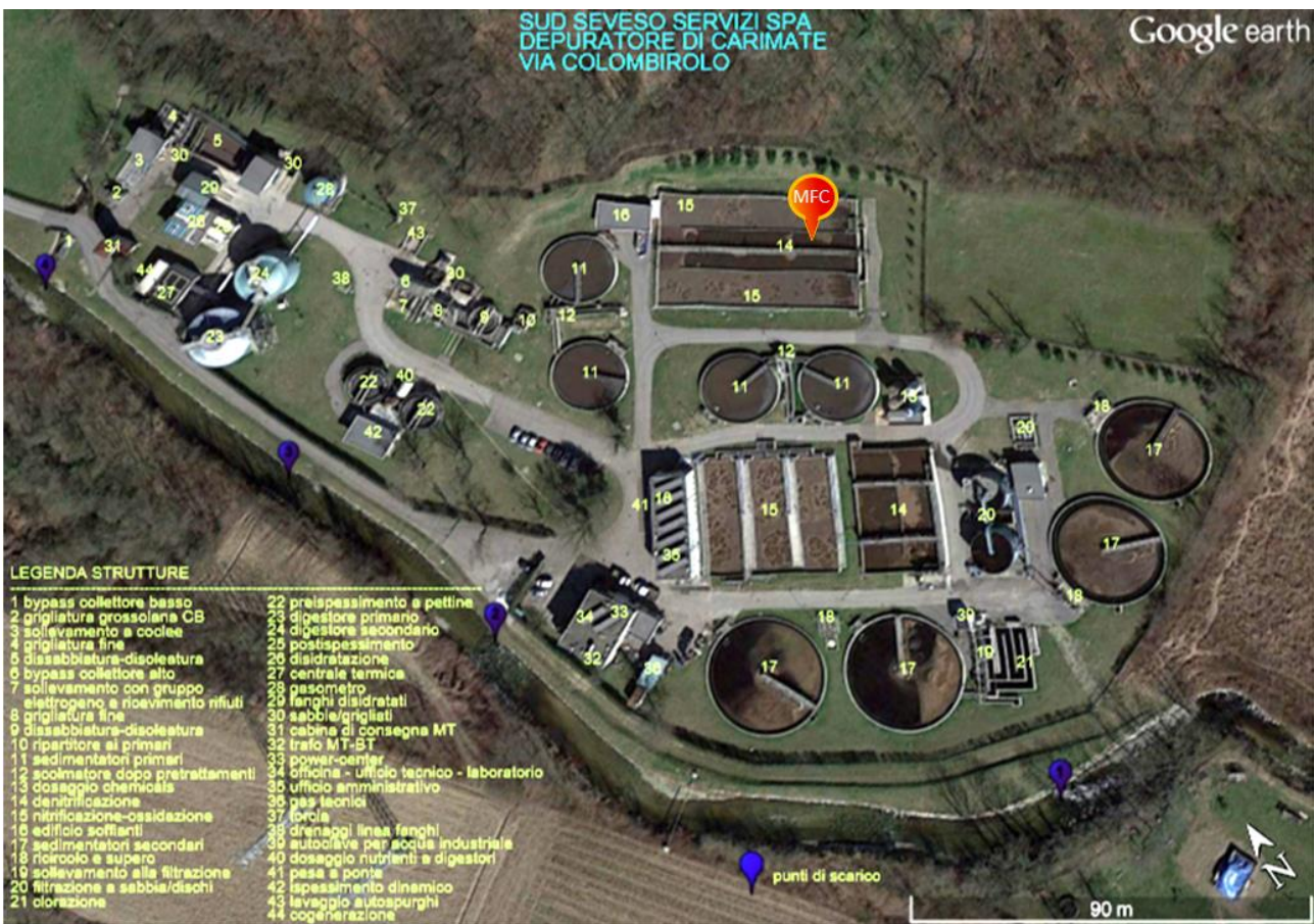
Figure 32 – Pictures taken during the field trials A) and B), map of the wastewater treatment plant of Carimate (CO) C). The exact point in the denitrification tank where the cells were placed is indicated with a red pointer.
