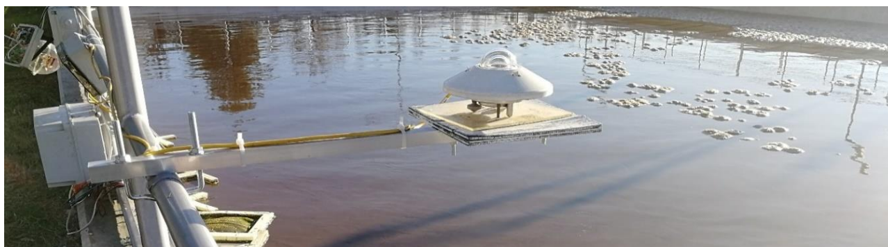
Figure 40 – Pyranometer placed over the denitrification tank of the wastewater treatment plant
