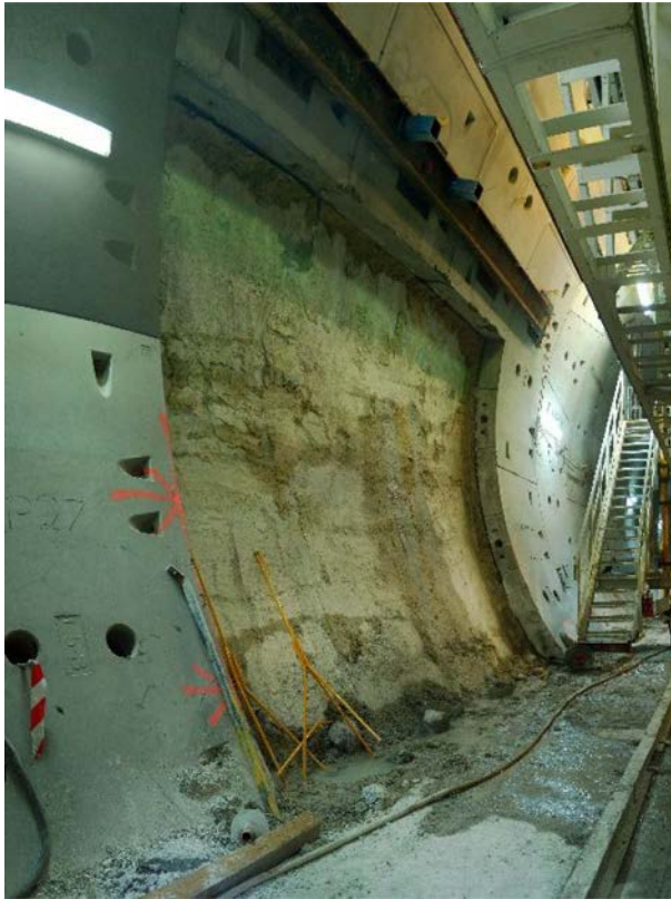
Fig. 4.6. An example of lining breakout from the Brisbane Airport Link, Australia (Arup).
