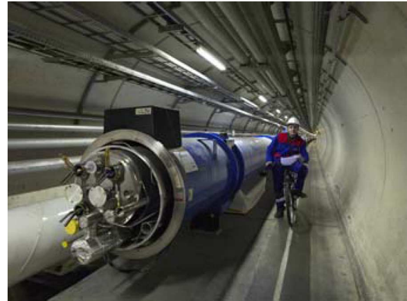
Fig. 1. View of the LHC ring. The 17th July 2006 the 616th dipole is installed.
