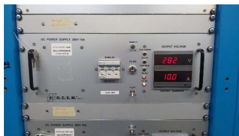
OCEM – USA15 ( V_{out} = 280V DC)
