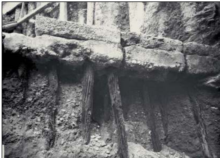
26 Via Cardinal Caprara, ponte (AFS D00794).
