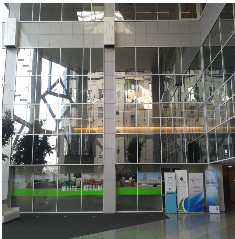
Figure 16. IMI Headquarters, Ixelles, Brussels, Belgium.
