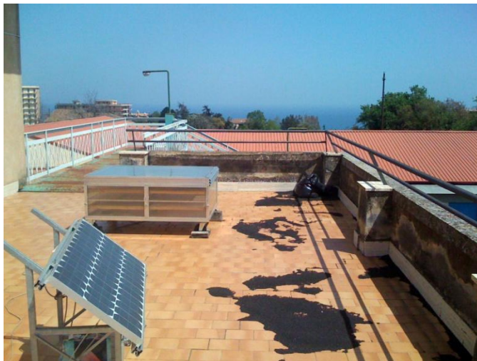
Fig. 6. A view of the solar drier system working at CRA-ACM in Acireale (CT).
