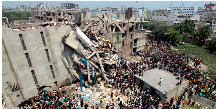
Picture-8: Collapsed factory building (Rana Plaza at Savar)
