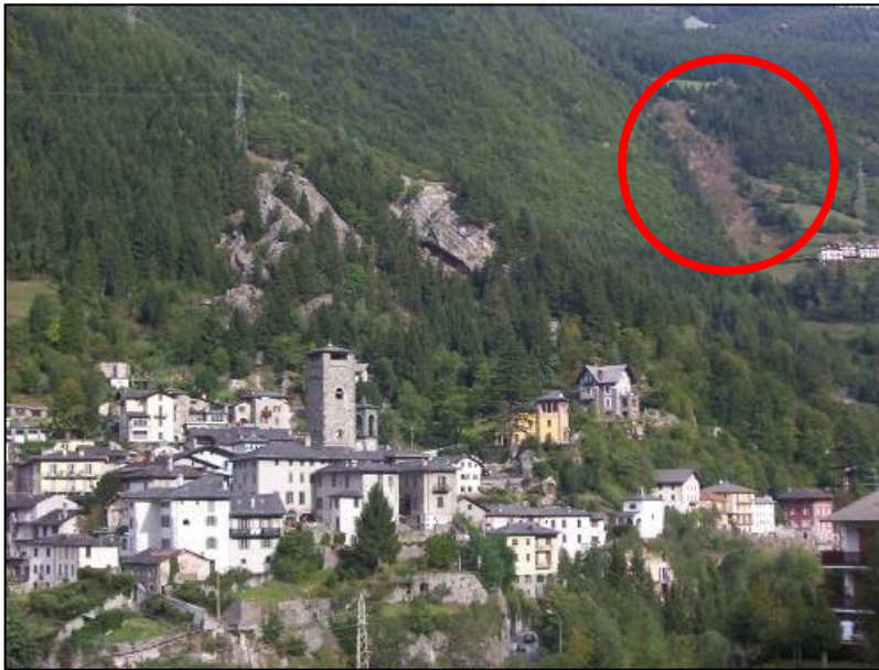
Fig. 5.4: Coren del Cuci waste-rock dump, located very close to Ripa locality; in foreground , Gromo village.
