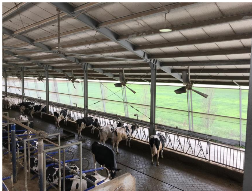
Figure 6. Cooling system applied in an Italian dairy farm equipped with high-speed fans and low-pressure foggers.
