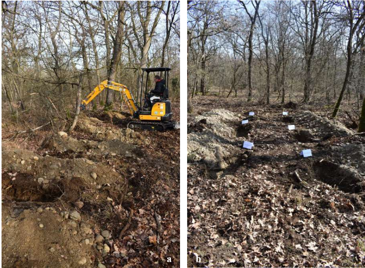
Figure 2.2: Pictures of the realization of the experimental burials at Ticino-LEAFs. a- on the left the mini excavator is digging the graves of group “GC”; b- on the right the group “GW”.
