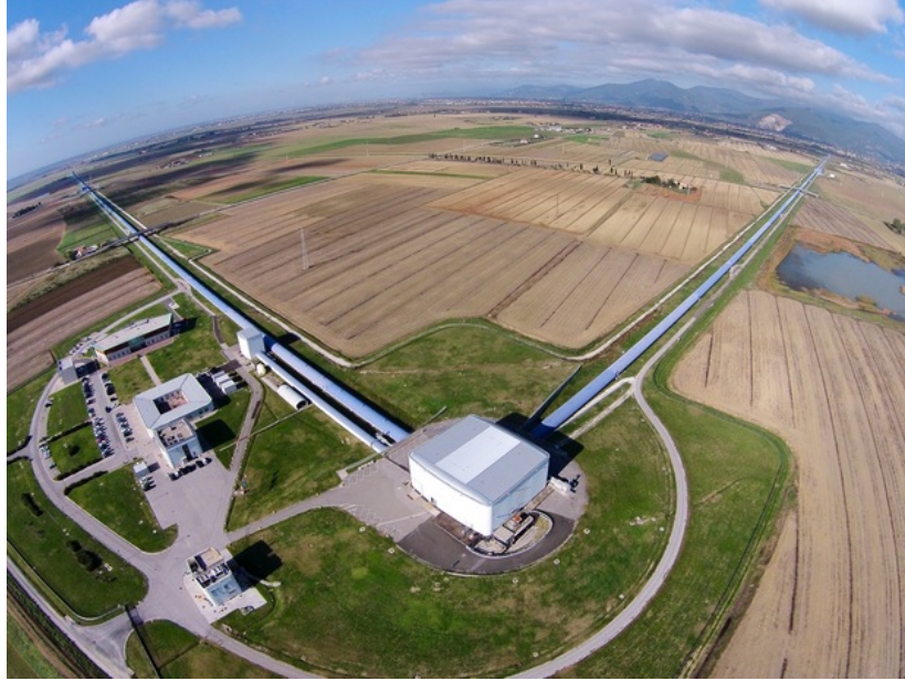
Figure 7.5: Aerial view of the Virgo site from https://www.ligo.caltech.edu .
