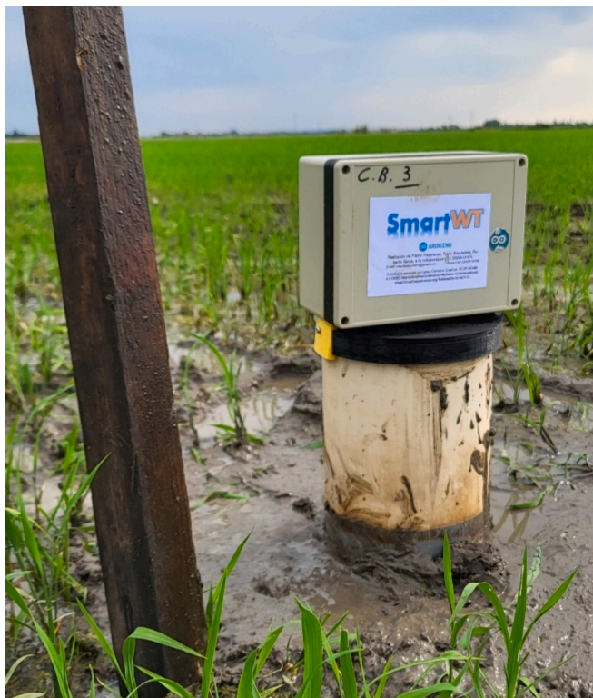
Fig. 3. Picture of one of the field installations (short pipes) made at the end of May 2024, after rice emergence, in Robbio (PV), Italy.
