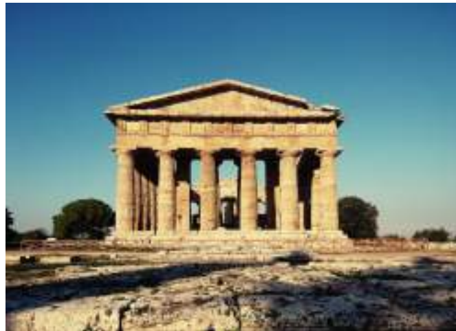
Figure 4. The view of the temple from the east side: the front façade. Copyright © V. Di Marco (Source: Own work CC BY-SA 4.0. Link: https://commons.wikimedia.org/w/index.php?curid=71188205 ).
