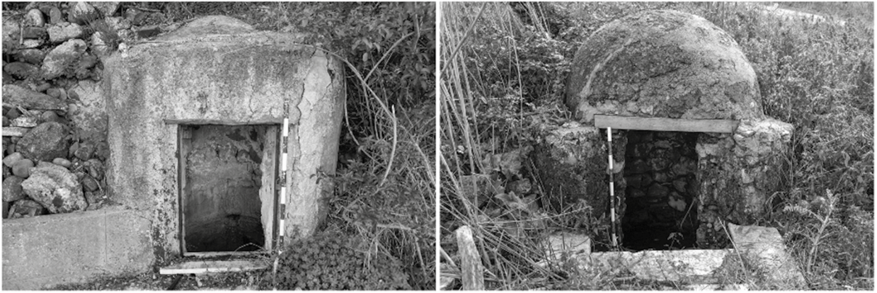
Figure 4 – Hydraulic elements: Cuba in Contrada Pioppo and Calemici
