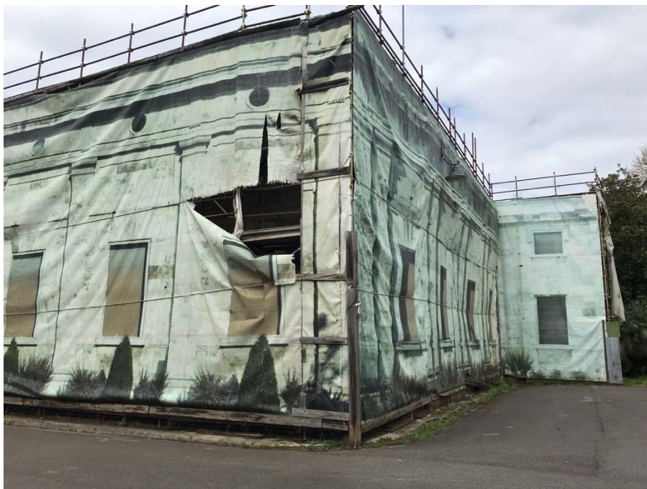
Figure 2. Scaffolding with a torn screen, Montecatini Terme, Italy, 2019. From author's personal collection.
