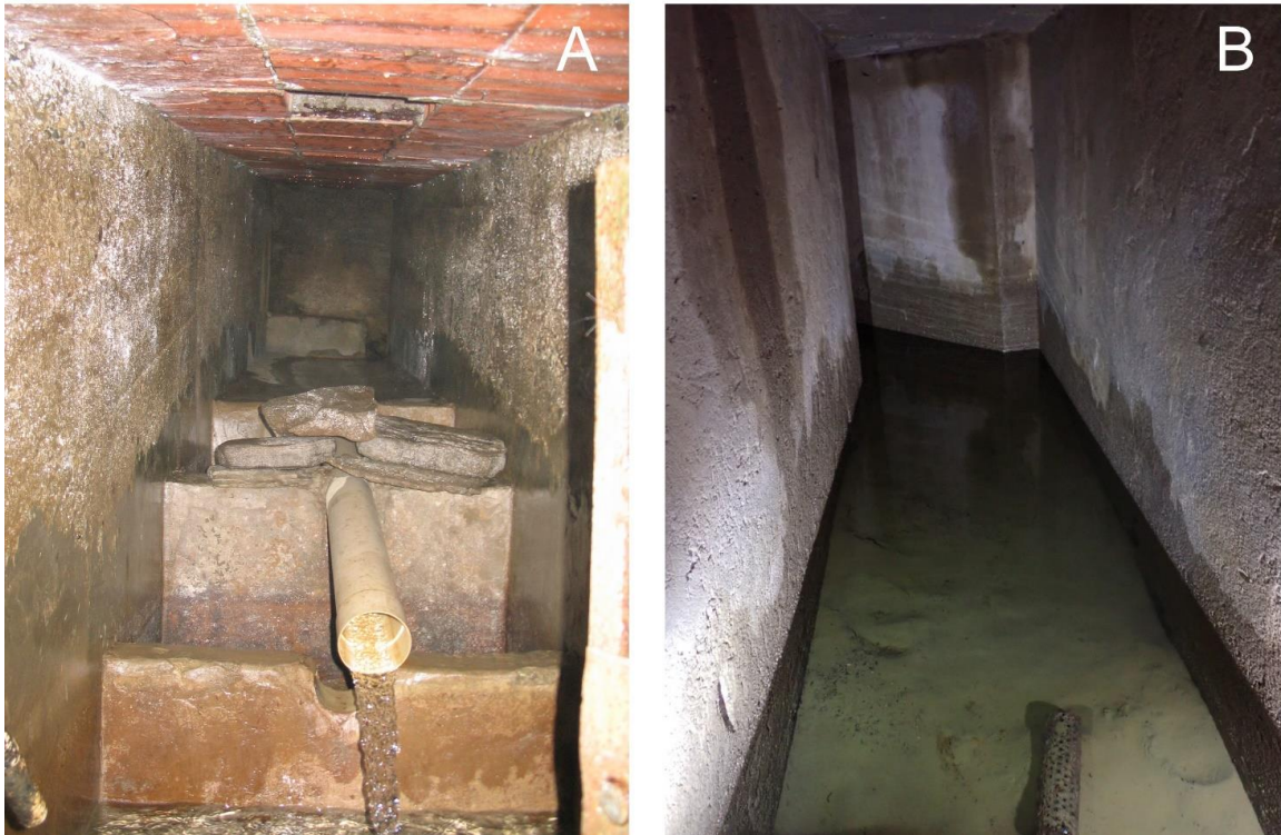
Figure 1. Sites of collection of Niphargus thuringius amphipods used during the experiment. (A) Short draining gallery in the locality of Valle Tolsera, Airuno municipality (Lecco, Northern Italy). (B) “Bottino di presa” in the municipality of Castello di Brianza (Lecco, Northern Italy).
