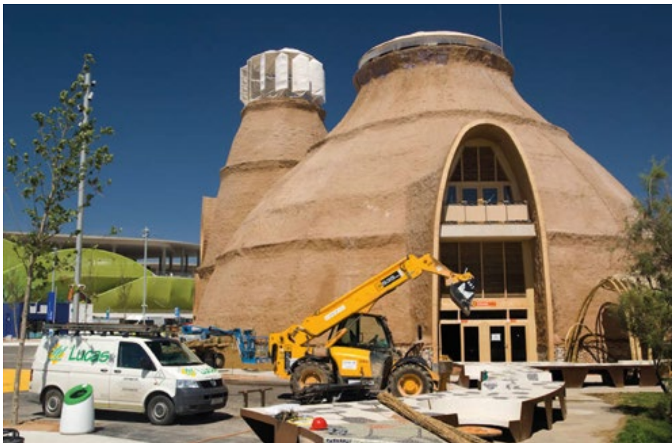
Final construction work on El Faro
