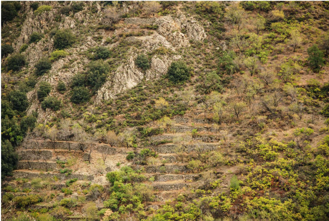
Figure 2. Unmaintained and collapsing dry-stone terraces in Polystipos community
