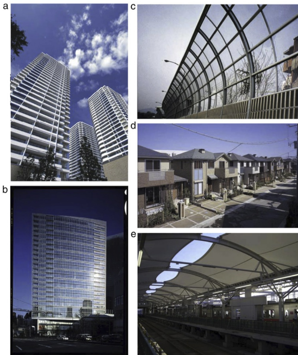
Figure A.7: Applications of self-cleaning exterior building materials. a Picture of the MM Towers, in Yokohama, coated with self-cleaning tiles (courtesy of TOTO). b Picture of the Matsushita Denso building covered with self-cleaning glass (courtesy of Nippon Sheet Glass). c Picture of the self-cleaning sound-proof wall (courtesy of Sekisui). d Eco-life-type houses using self-cleaning tiles and glass (courtesy of PanaHome). e Self-cleaning roof of a train station in Motosumiyoshi (courtesy of Taiyo Kogyo). Reprinted from Surf. Sci. Rep. , Vol. 63, A. Fujishima et al., \text{TiO}_2 photocatalysis and related surface phenomena, pp. 515-582 [1] Copyright 2005 with permission from Elsevier.
