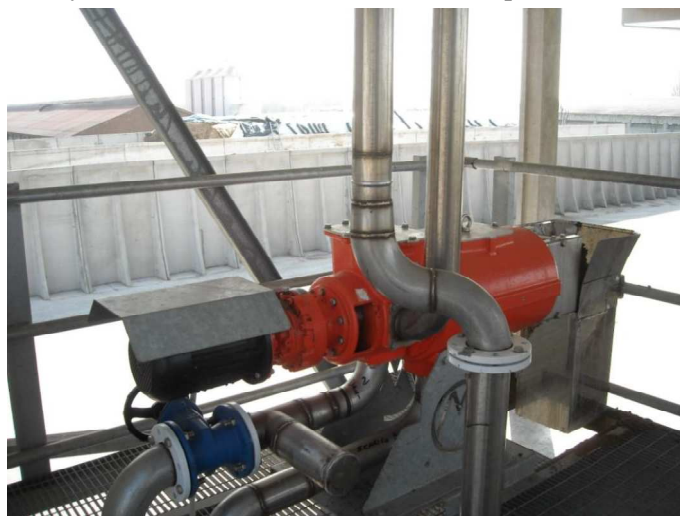
Figure 2.3. Screw press separator (FAN PSS 3.2)
