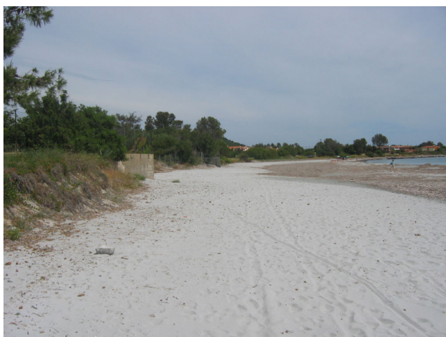
Figure 3.94 - Northern sector and buildings close to the beach (May 2010).
