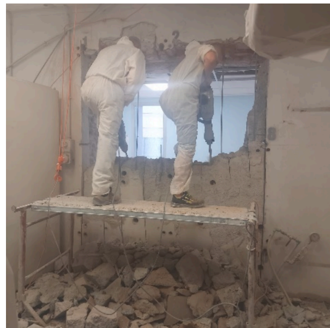
Fig. 10. The demolition of the wall.
