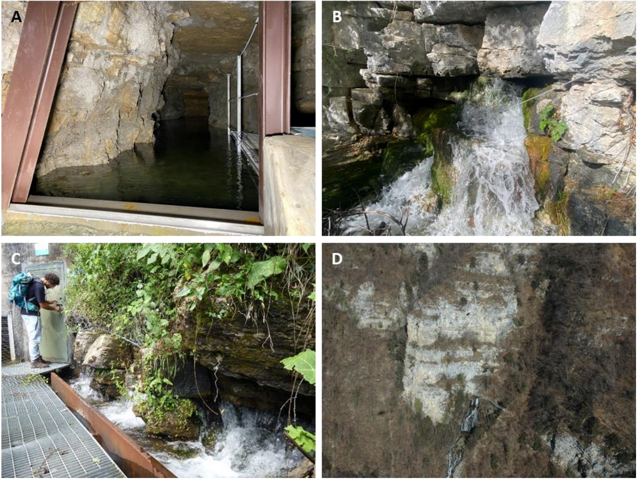
Fig. 2.9 A: Acqua Bianca water collection tank. B-C: water overflow from the rock layers. D: top-down view of the Acqua Bianca waterfall.
