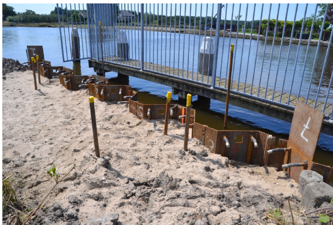
Fig. 7. Energy quay wall sheet pile installation. Heat exchanger pipes are observed above the ground surface attached to the sheet piles ready to be connected. Vertical pipes are part of the instrumentation system.
