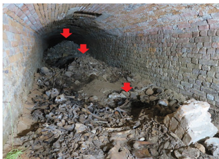
FIGURE 4. Anthropic conoid accumulations discovered right below the square manholes located on the vault of chamber “O” (Courtesy of Belgiovine and Capuzzo 2021).
