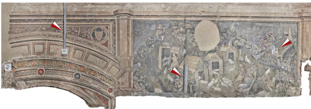
Figure 1 Dense point cloud with the texture of the residual traces of metal poles.
